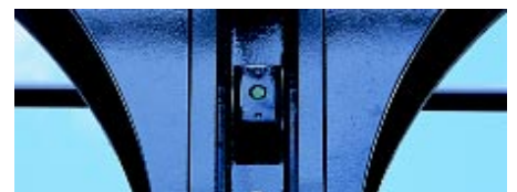
One of two PE Sensors that automatically operate all 21 towers at sunset.
